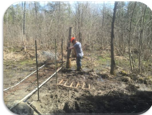
Fence and gate repair Summerstown Forest, Township of South Glengarry
