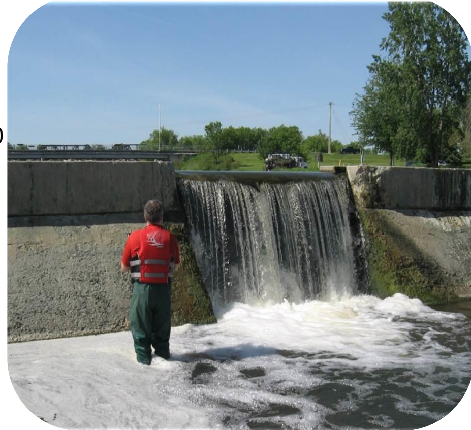
Casselman Weir Repair Village of Casselman
