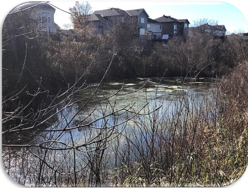
Radison Stormwater management facility Russell Township
