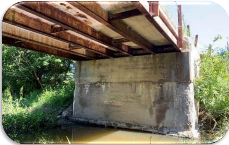
Butternut Creek Bridge to be replaced, Nation
