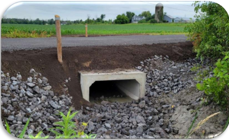
Devereaux Road emergency culvert repair, Ottawa
