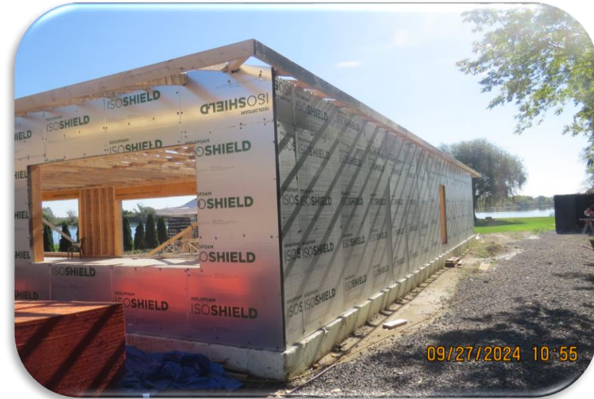
Permit compliance inspection Municipality of South Dundas
