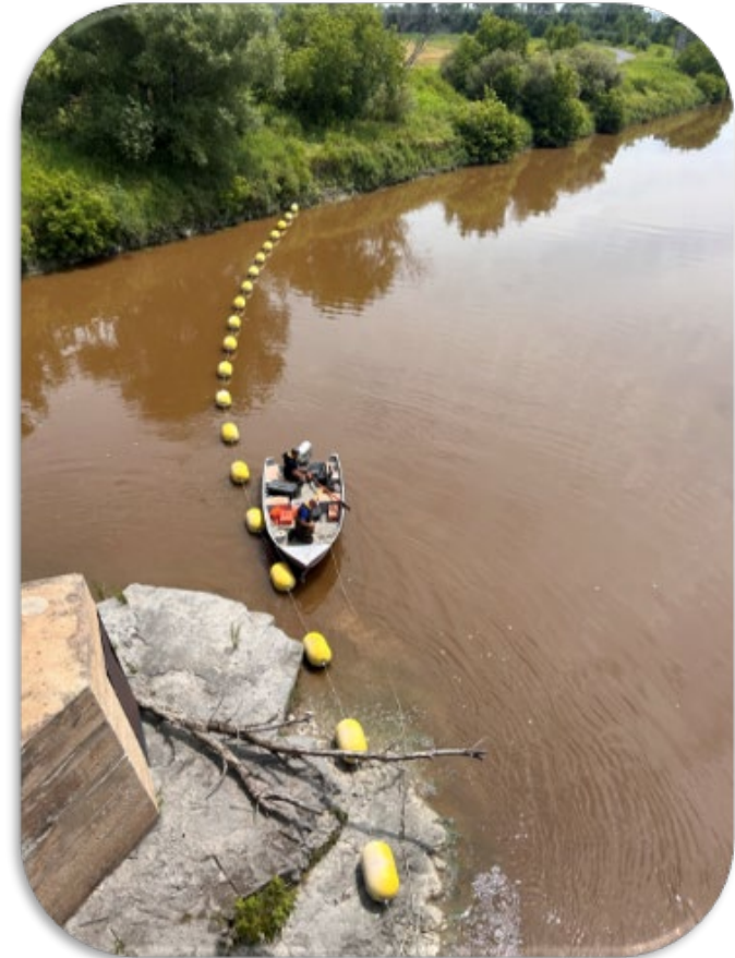
Plantagenet Weir Safety Boom Township of Alfred and Plantagenet
