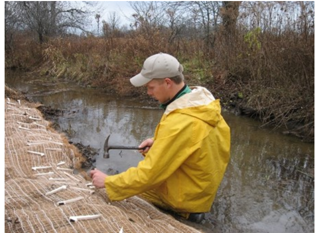
Stabilizing banks with straw mats
