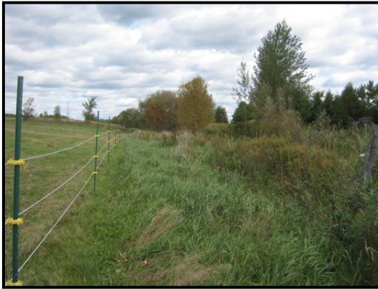
Cattle fencing and alternate watering project site for WEBs project.
