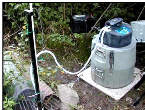
Figure 2: Automated sampler set-up to sample flow from the tiles for the WEBS – controlled drainage BMP.
