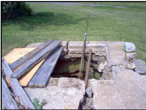
An example of an abandoned well that is being decommissioned with the EOWRC funding.
