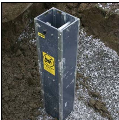
Figure 1: Tile drain control structure installed on a tile header for the WEBS – controlled drainage BMP.
