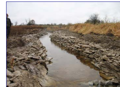
This picture was taken on October 23, 2006 after six volunteers worked hard all day placing by hand, the stones along the fish passage located at Indian Creek, West of the village of Spencerville.
