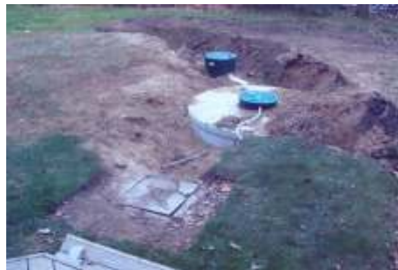
“After” septic system replacement, prior to final site grading.
