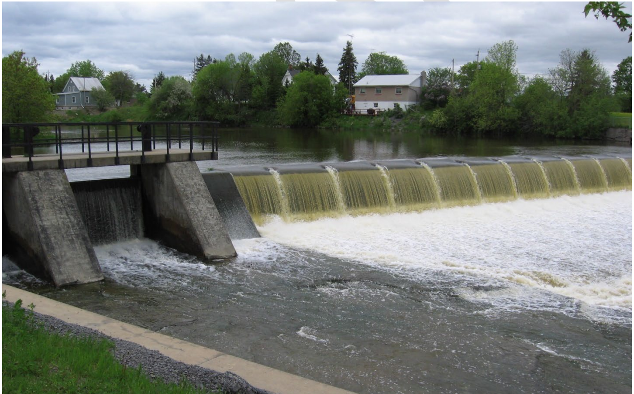
Figure 18. Crysler Dam photo in Crysler, Ontario.
