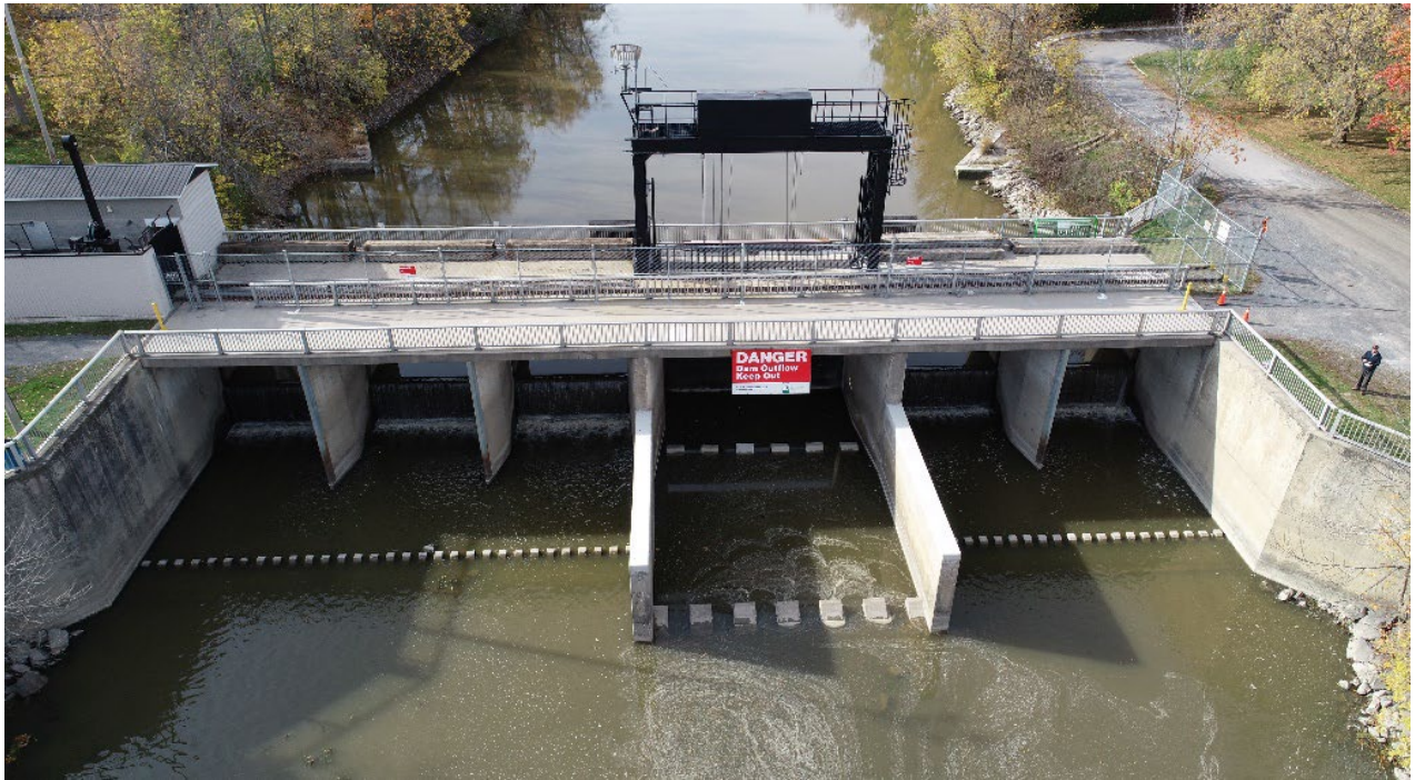
Figure 17. Chesterville Dam photo in Chesterville, Ontario.
